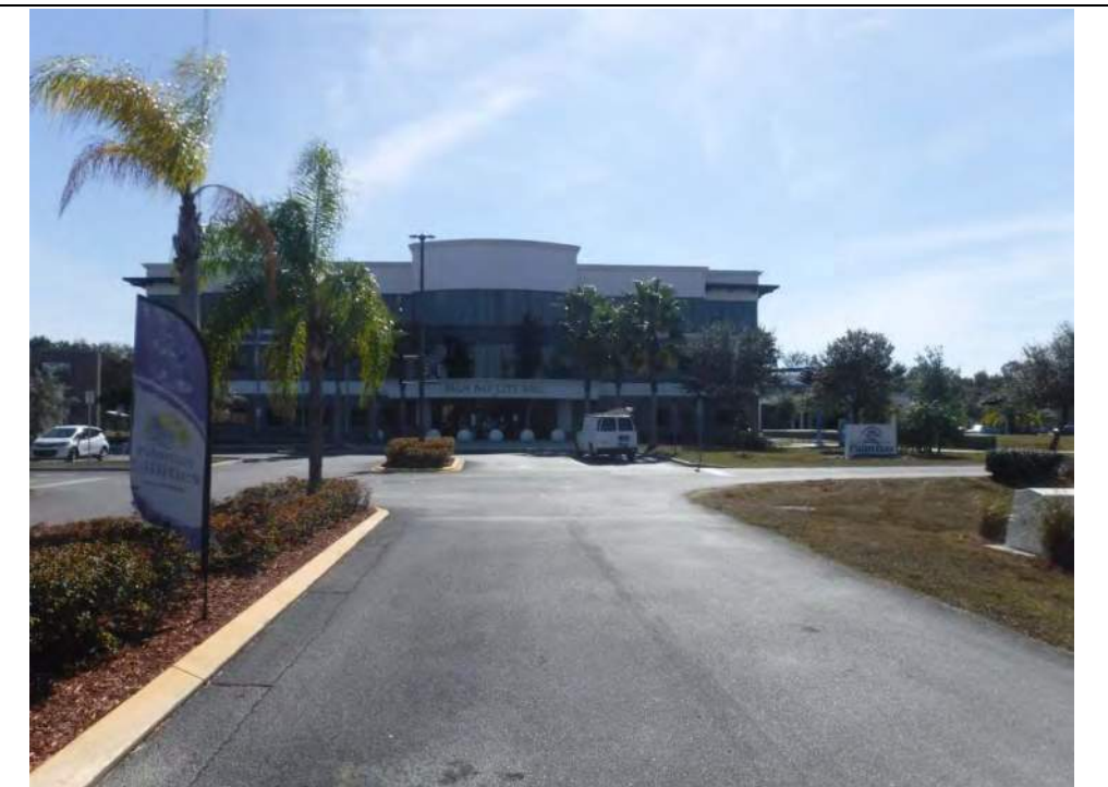
Photo taken from northeast of the site facing southwest. The Palm Bay City Hall is visible.
