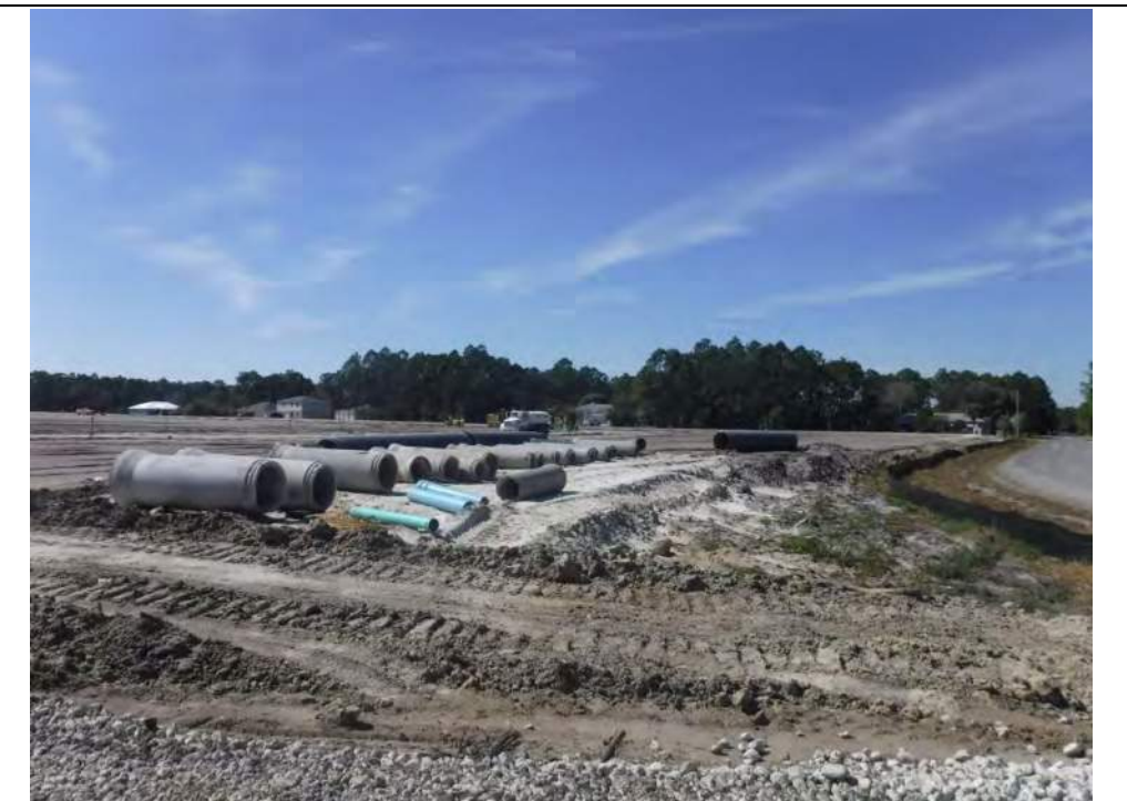
Photo taken from north of the site facing south. The area is under construction and currently contains concrete and PVC pipes.
